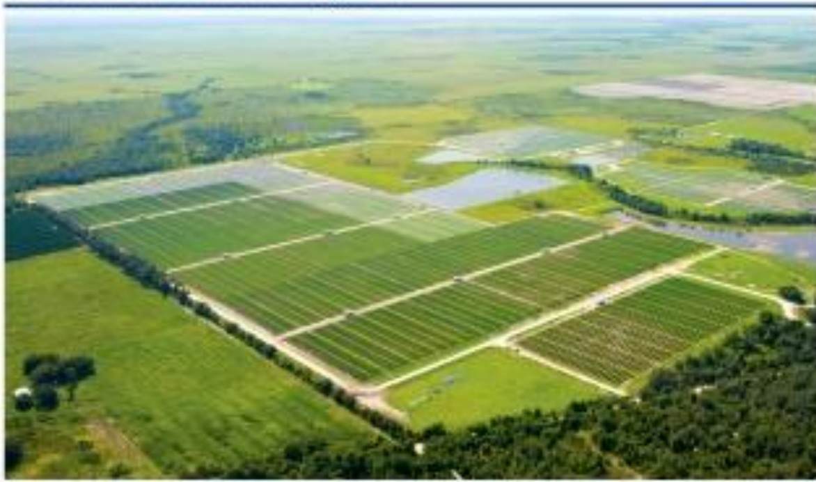
DeSoto Next Generation Solar Energy Center
